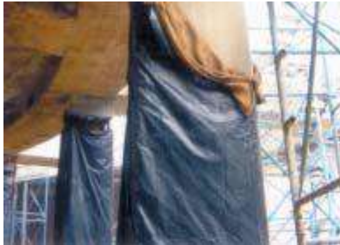
Curing vertical surface by wet covering.
