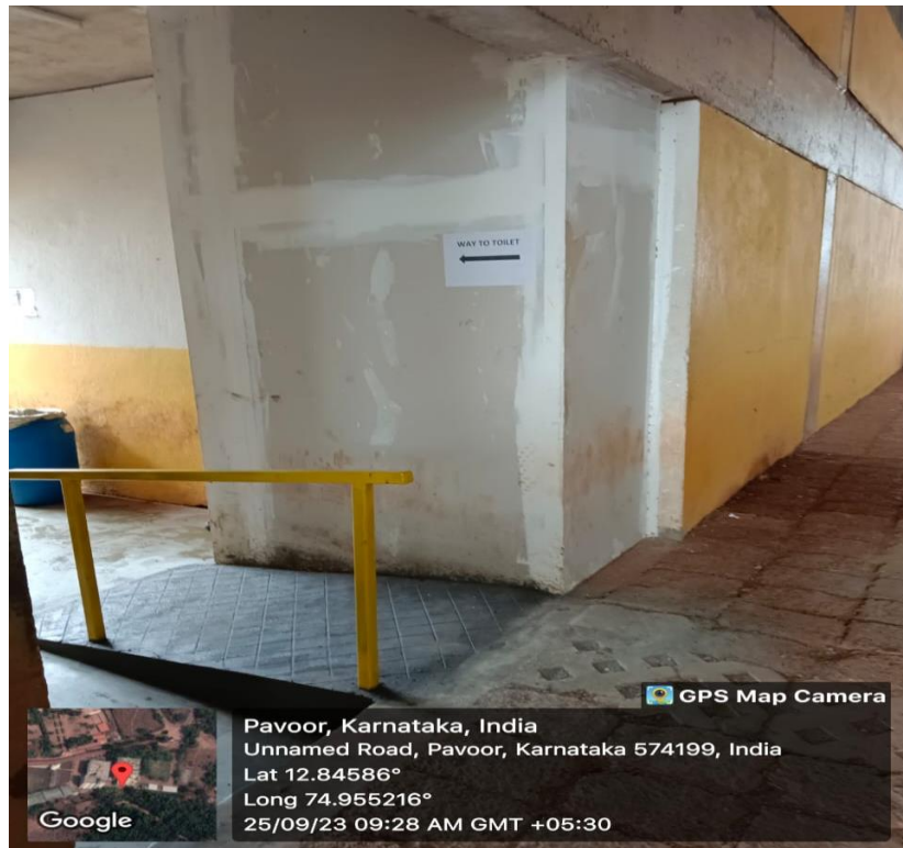
Fig. 5 Ramps with hand rail
