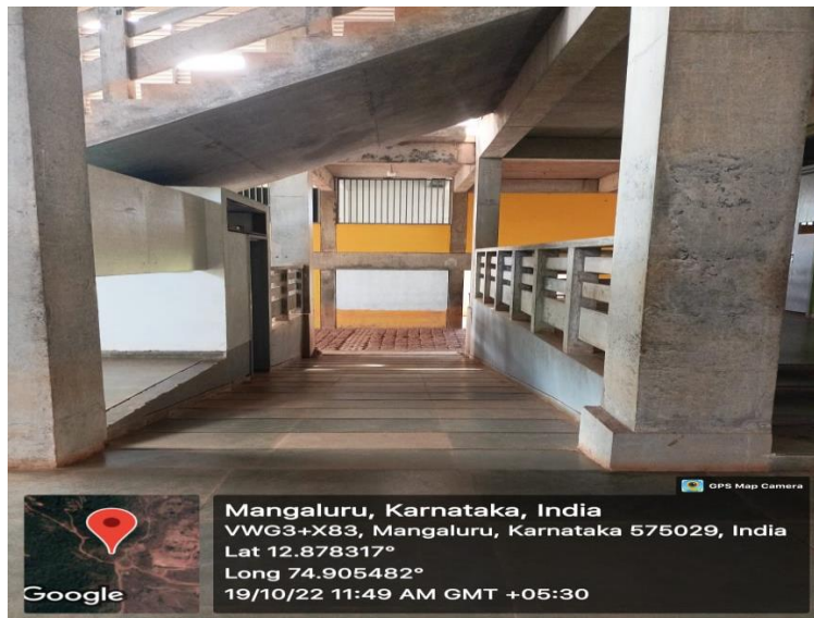
Fig.1 Ramp near the Entrance
