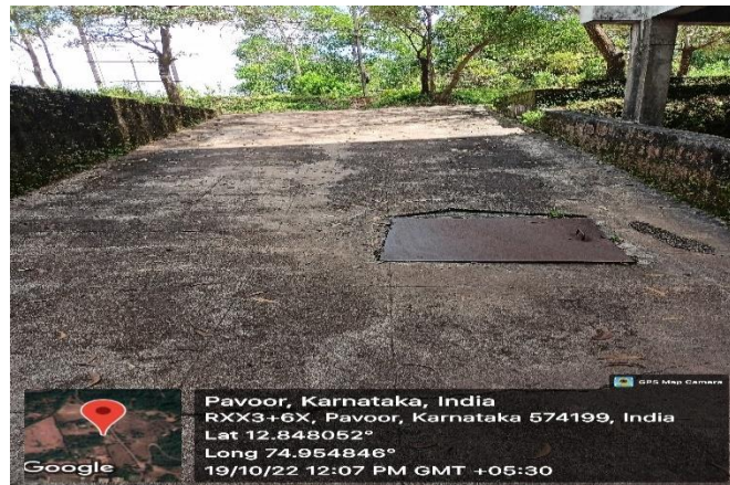
Fig. 7 Slope provided towards the sump
