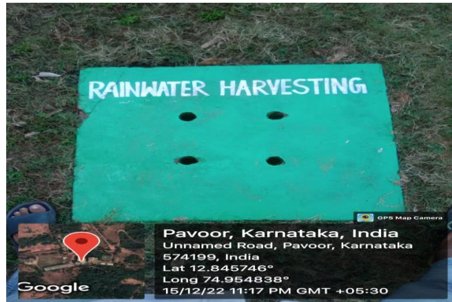
Fig. 4 Recharge well No.3 in the Arena
