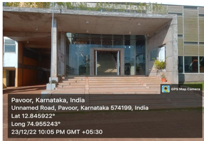
Fig.2: BIT Reception desk , Passage and Front view of BIT
